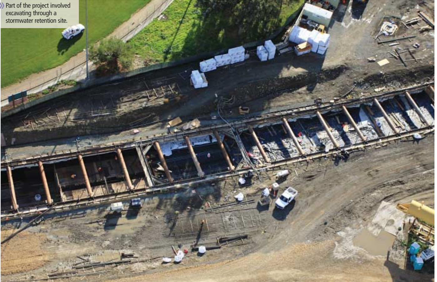
To form the walls, crews are using a travelling concrete forming system developed by vendor EFCO. The form system is hydraulic and self-driven, which allows sections of the walls and deck to be formed monolithically and faster than conventional forming methods, Majors and project engineer Mike Wathen say.
